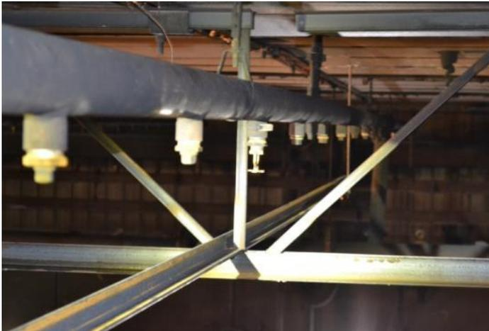
Figure 1. 22-inch Deep Bar Joist with Bridging Member.
