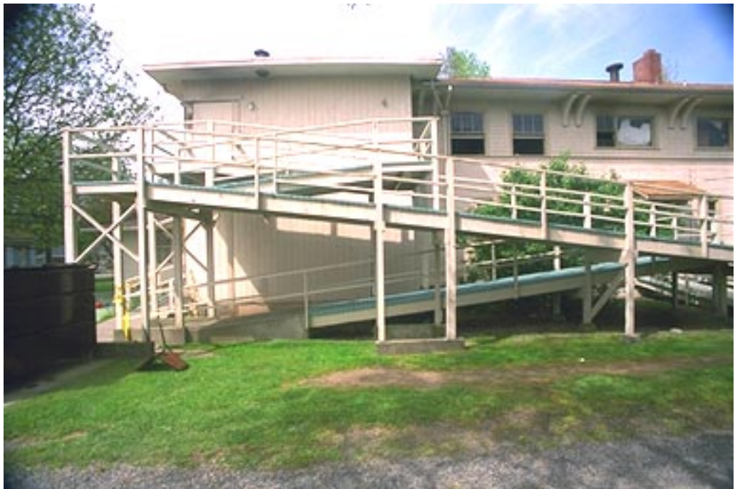
Photo 3. This ramp provided an exit path from the second floor.
