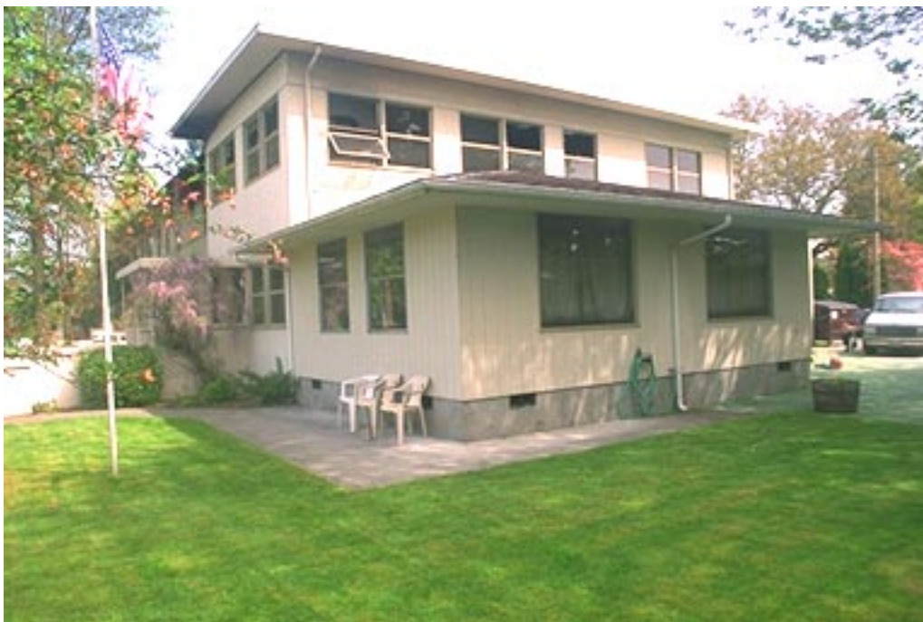
Photo 1. The southeast corner of the facility.
