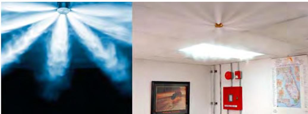
*Figure 3: Example of Clean Agent System Discharge (<http://www.arafire.com.au/fire-suppression-systems.htm>)*
