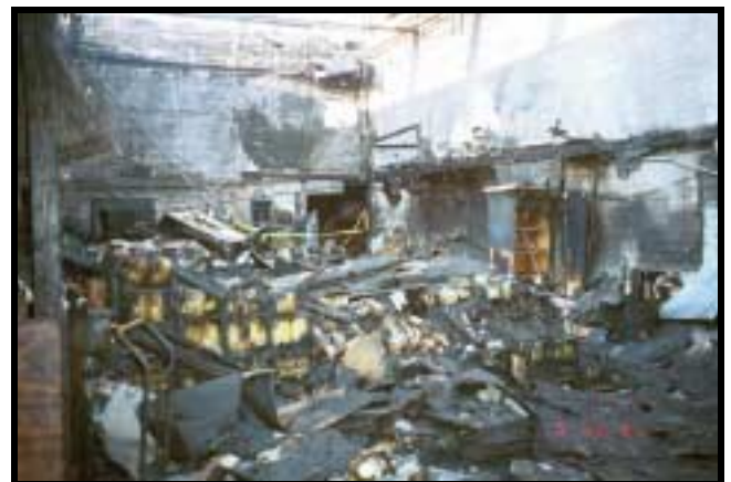
View of supermarket stock room (NFPA)
