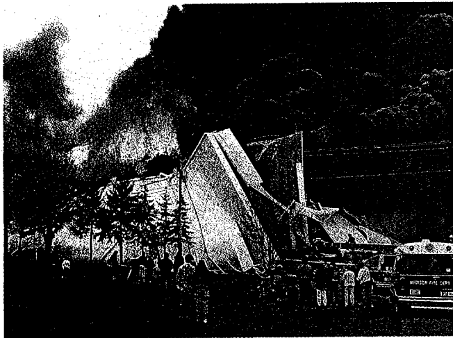
The foam insulation contained in Freezer 8's walls, partitions, and roof generated heavy black smoke as it burned. This photograph was taken from the northeast corner of Freezer 8.
