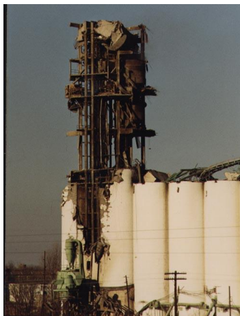
Figure 6 - Inland Concrete Head House Damaged From An Explosion
