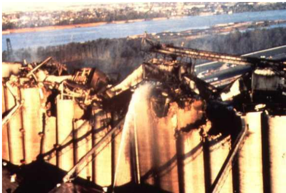
Figure 1 - Westwego, LA Explosion 12/77
